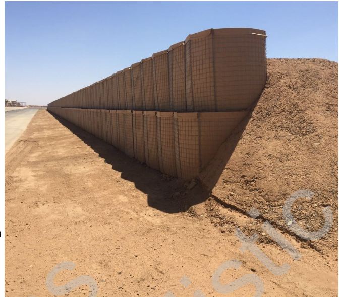
Fig. 1: Defensive barriers, constructed from DEFENCELL MAC™
