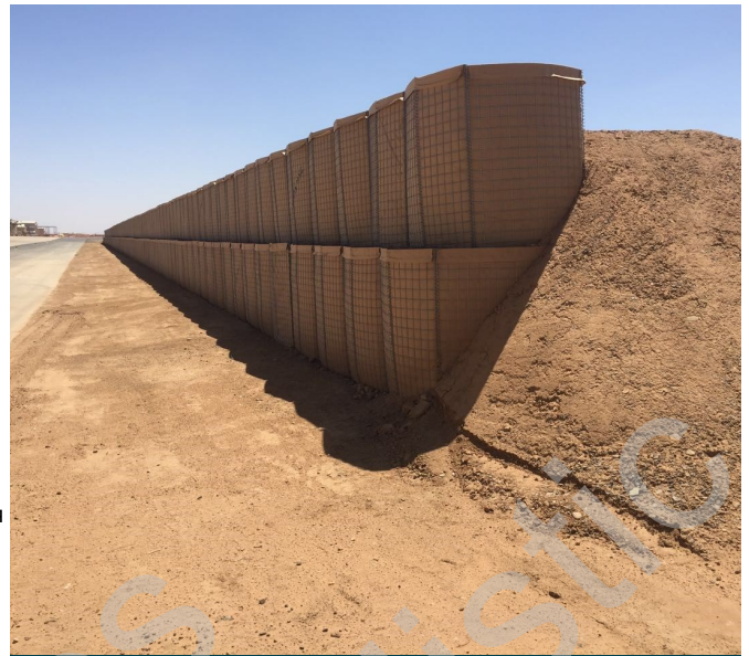
Fig. 1: Defensive barriers, constructed from DEFENCELL MAC™
